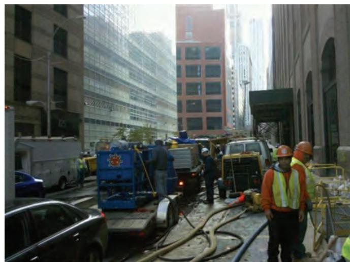
**T&T Marine Hydraulic Power Unit With Discharge And Hydraulic Hoses With Equipment On Stake Truck**
